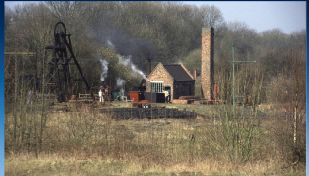
The Racecourse Colliery at the Black Country Museum. This mine is very similar to the other 499-599 small-pit coal mines/colliers previously in operation in the Black Country.
